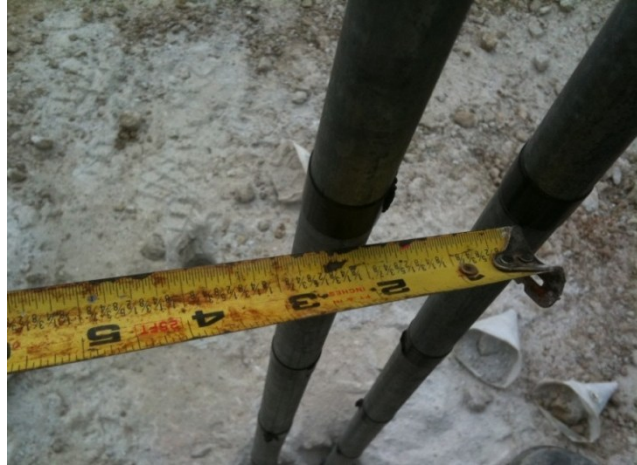
Figure 3-11: Measurement of Hole Deviation at Two Feet Above Ground Surface
